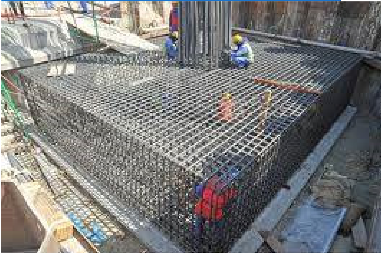
Steel fixing in progress at pile cap 4
