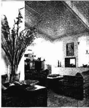
Seating placed directly below the beam is afflicted.
