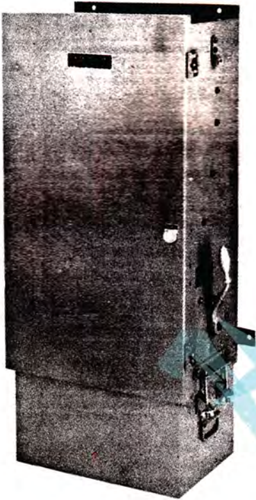
Fig (4-63) Autotransformer type manual starter.
