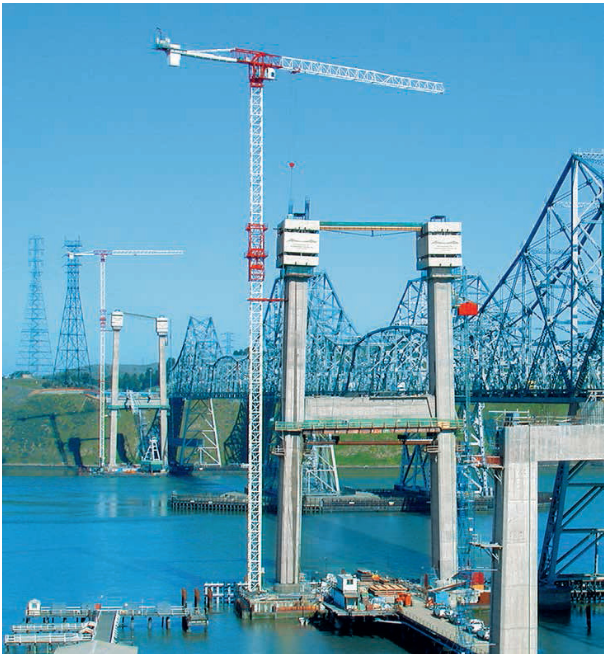
ပုံ(၅.၁၈) A mobile crane superstructure mounted atop a tower
