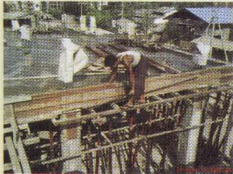
Removal of beam form
