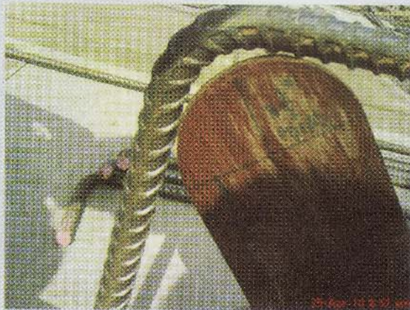
Checking the radius of a 90° hook
