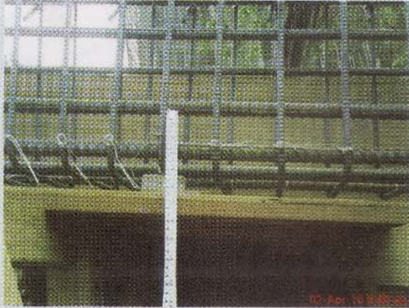
Checking the spacing between two layers of steel
