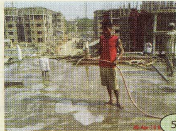
Spraying water to cure the slab
