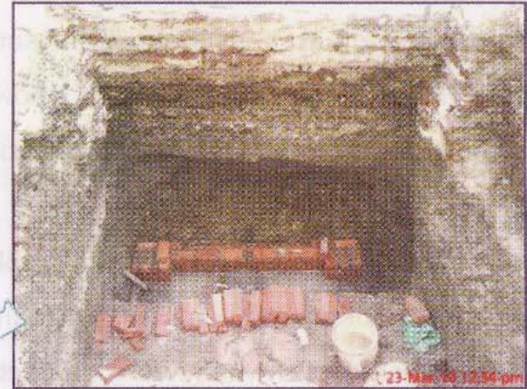
Caving-in of earth at basement excavations in poor soil
