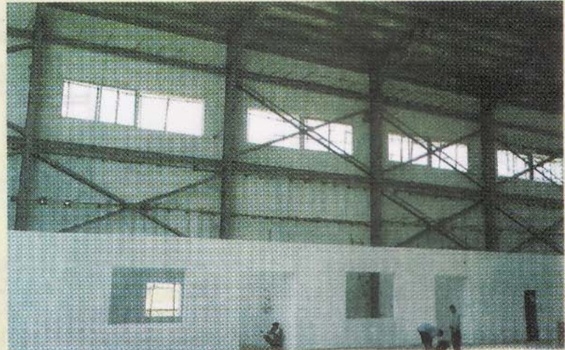
Column diagonal bracing
