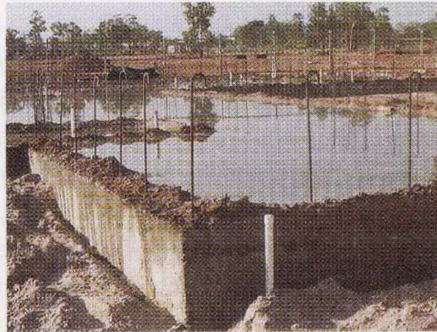
Concrete slab cured by ponding
