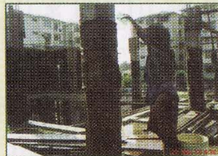
Wetting the gunny wrapped around the column
