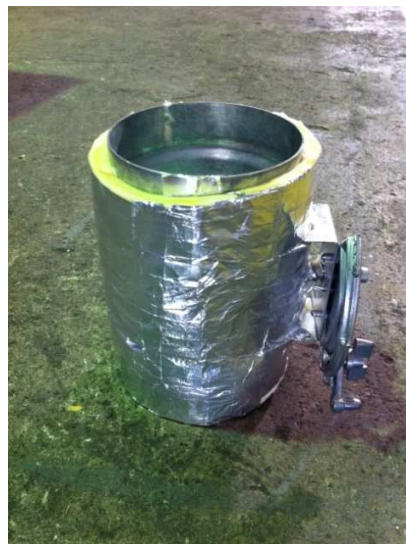
Figure 17. VCD with insulation
