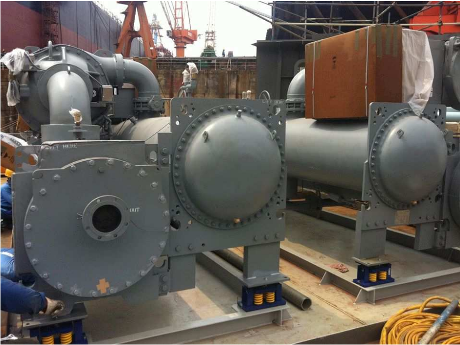
Figure 6. Fresh water cooled centrifugal chiller
