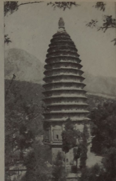
The 12-sided Songyue Pagoda in Henan, which was built in the sixth century, features close-set eaves.
