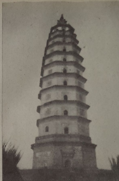
This tower-like Liaodi Pagoda in Hebei Province was erected in the 11th century. Standing at 84.2 meters (about 276 feet), it is the tallest pagoda in China.
