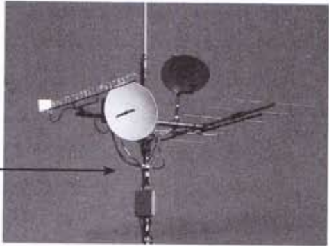
Television Repeater Antenna
