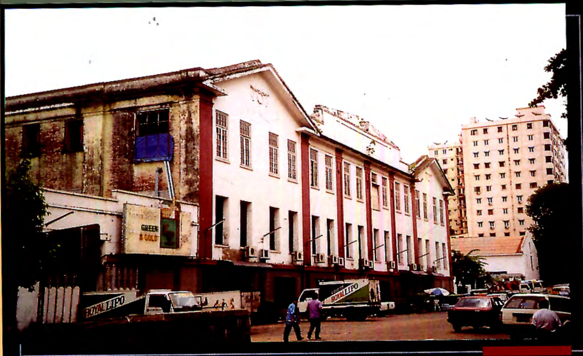
The building is nowadays holding a soft drink factory in Wadan Street.
