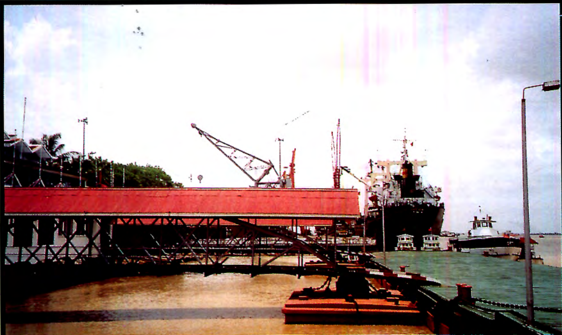
Unloading cargo at Nan Thida jetty in 2003
